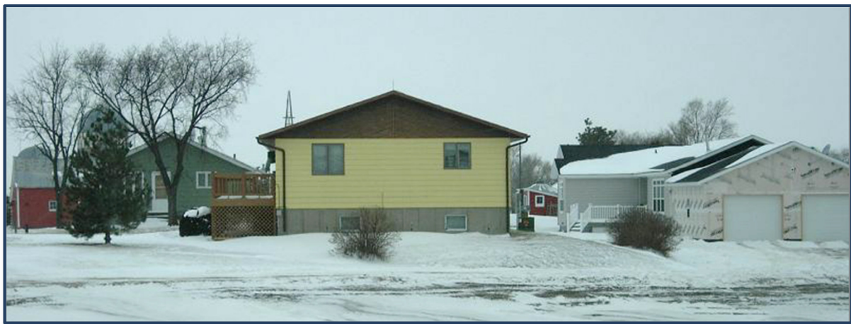
FIGURE 1 LOOKING WEST. BLUE HOME LOCATED ON FOUNDATION THAT IS PROPOSED TO BE USED FOR NEW STRUCTURE. TAKEN WHEN NORTHERNMOST HOME WAS BEING CONSTRUCTED.
